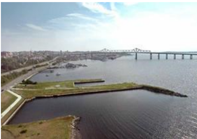
Above: An aerial view of the Fall River City Pier
