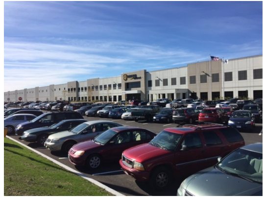
Above: Amazon project is complete and operational
