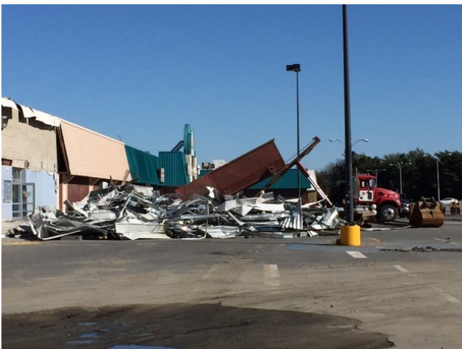
Above: Redevelopment of the New Harbour Mall underway
